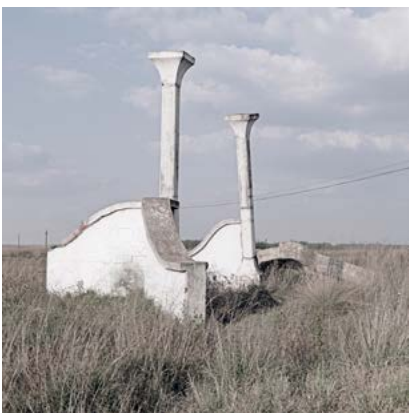
The remains of a abandoned farm entrance gate near an expanding township. Ermelo, South Africa, 2011
